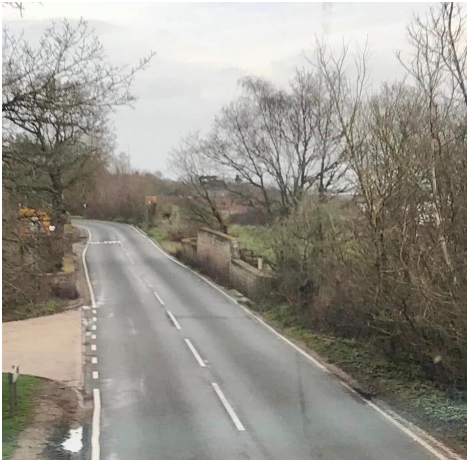
Alresford Road railway bridge. In the distance can be seen Marsh Farm Corner on Wivenhoe Road. February 19 th , 2024.
