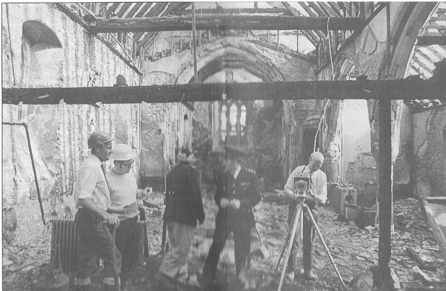
Figure 31 - St Peter's Church the day after the Fire, Sunday October 3 rd
